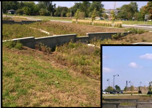
"Stepped" infiltration basin in Oakdale, MN.
